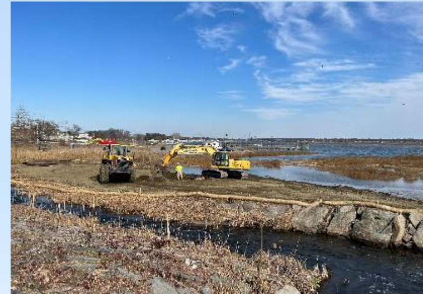
One Beacon Point – Excavation
