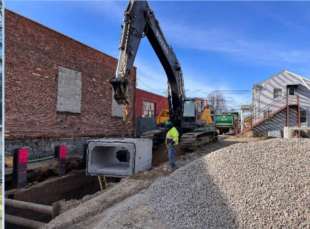
Box Culvert Installation
