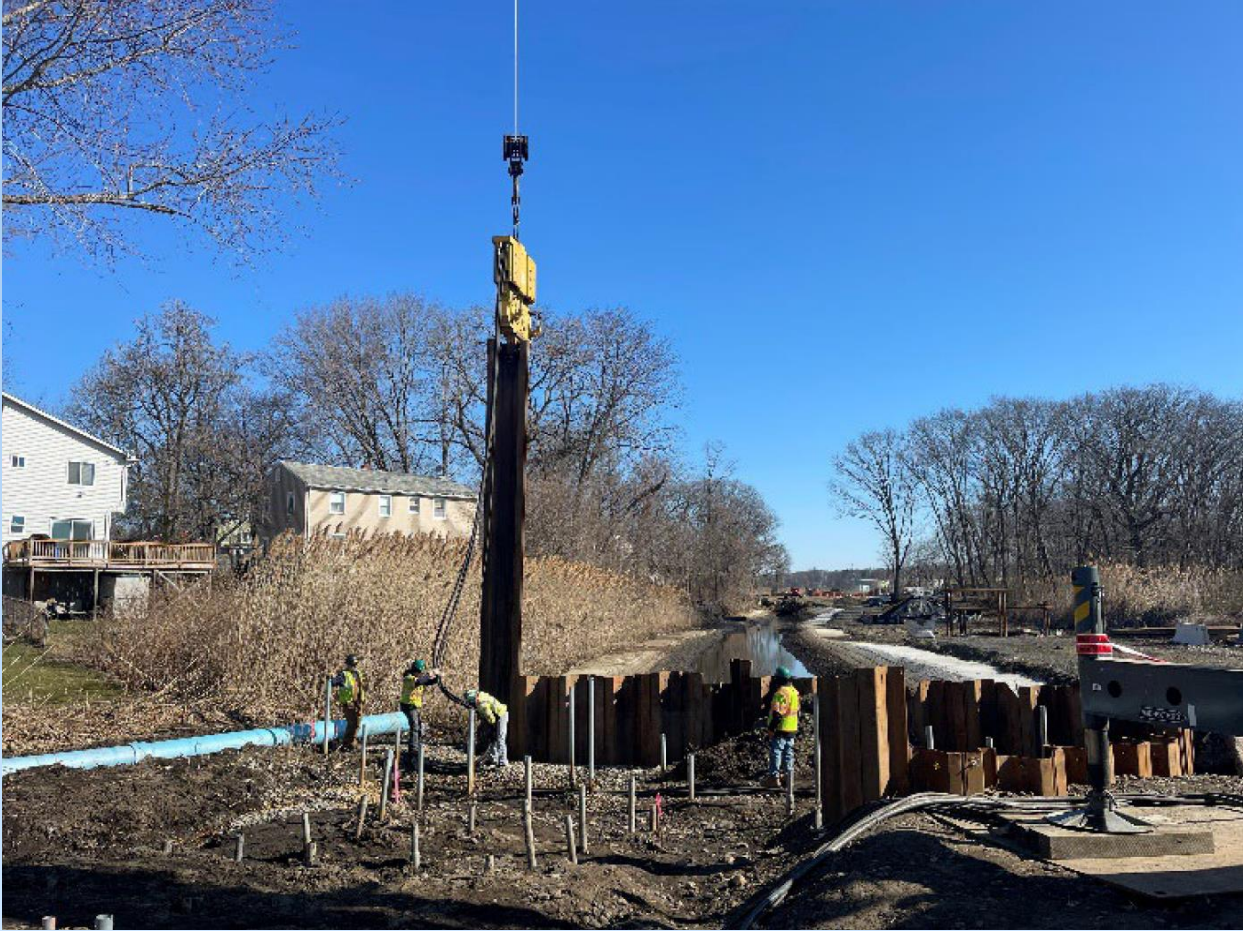
Sheet Pile Installation at Headwall
