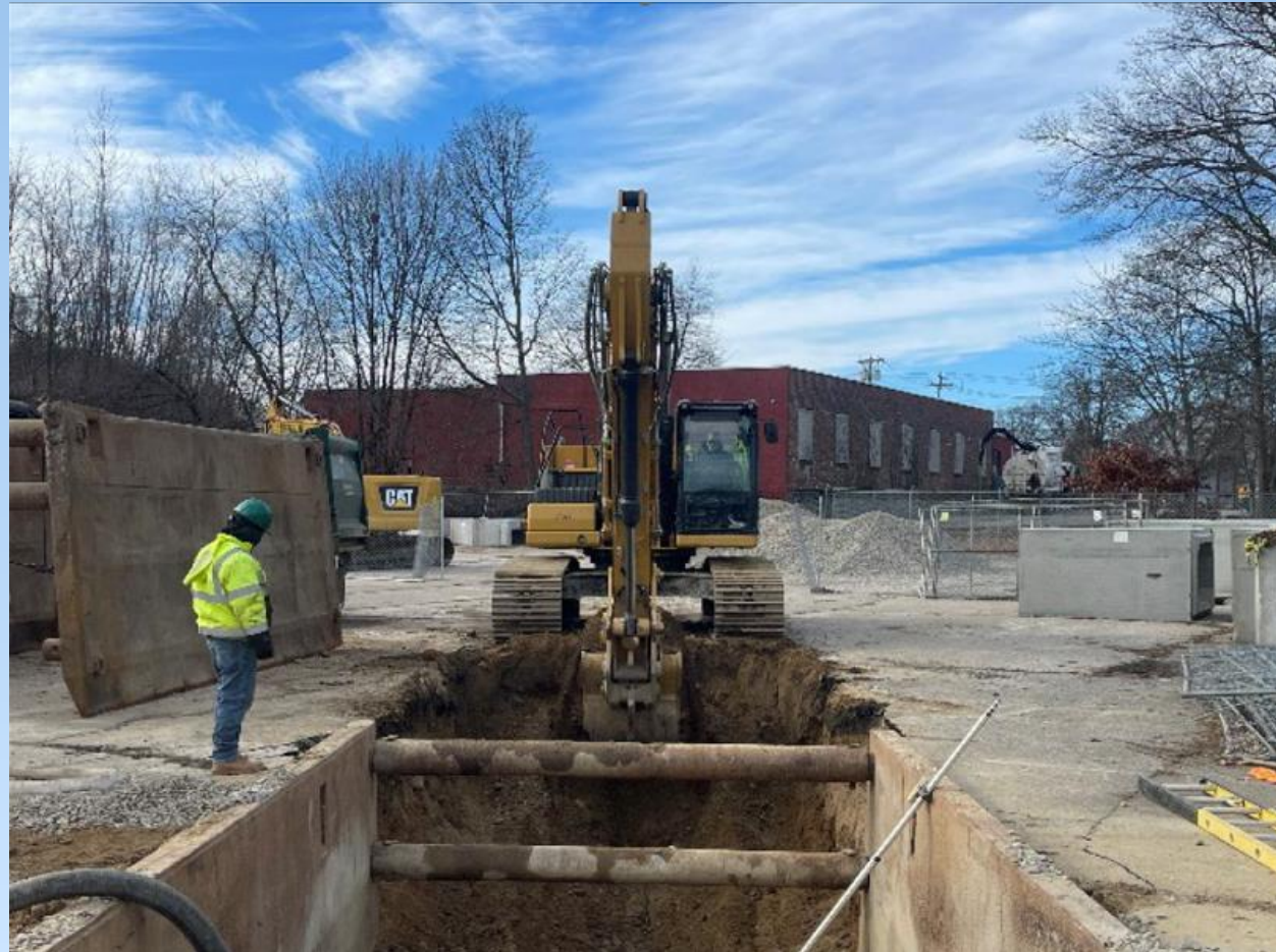
Trench Box for Culvert Installation
