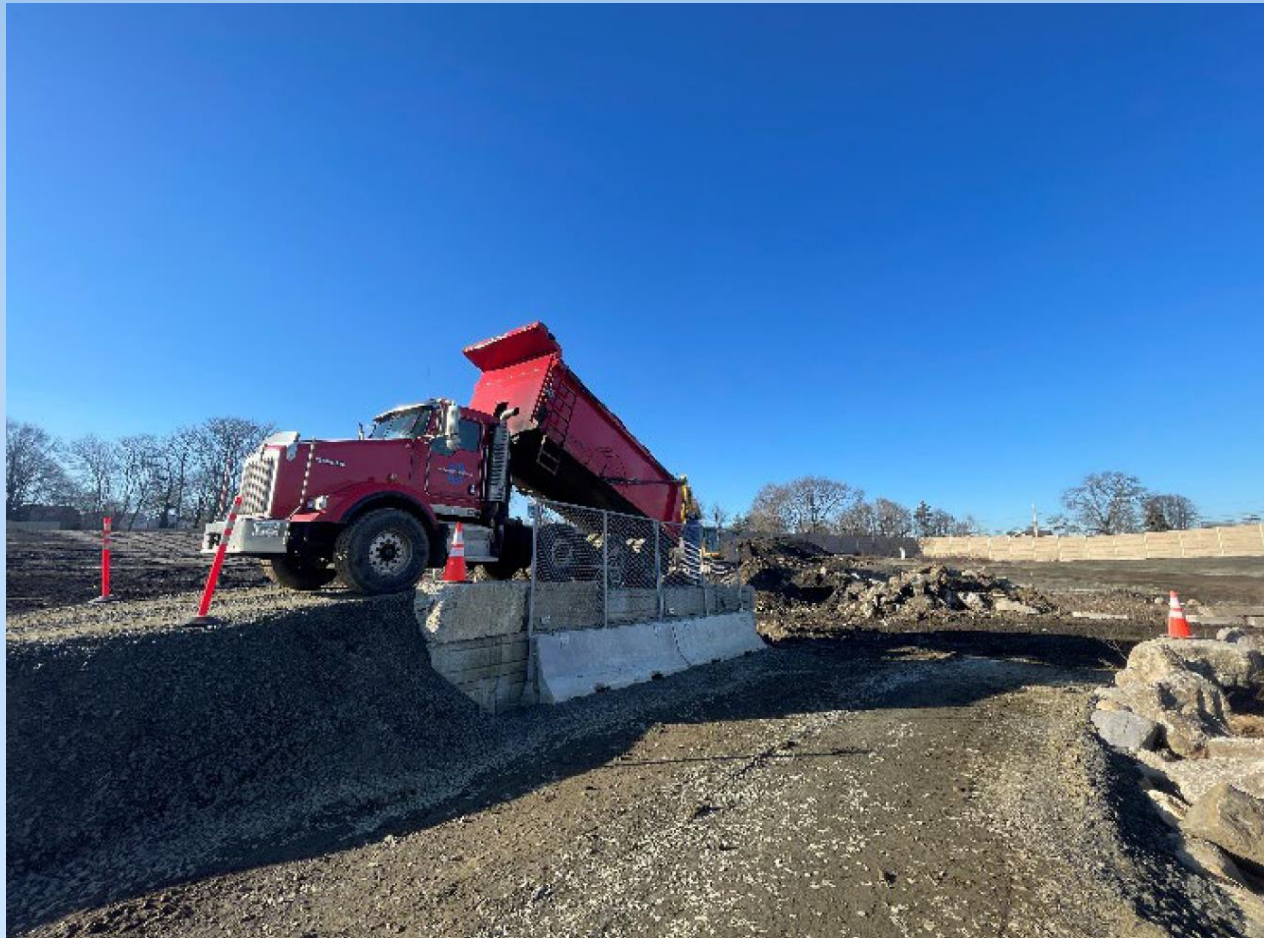
Material Placement Within OU4 Consolidation Area
