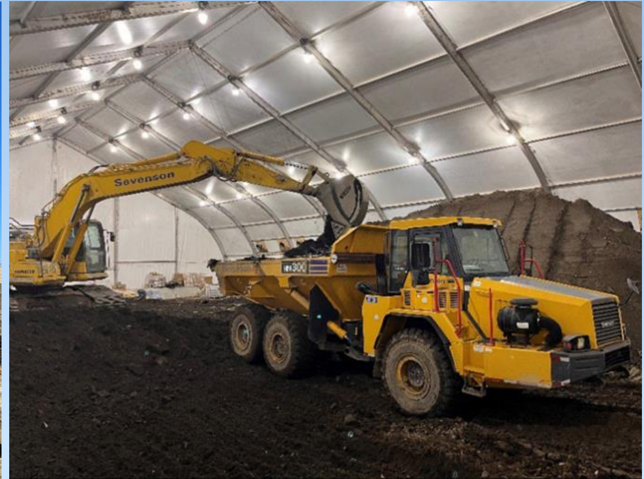
Loading Amended Soil for Consolidation
