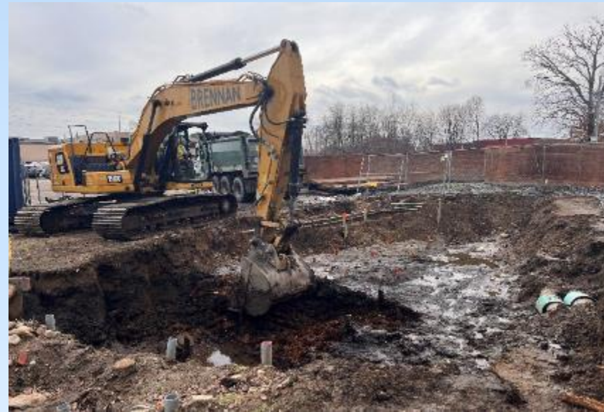
Stormwater Channel - Excavating to Pour Helical Pile Caps
