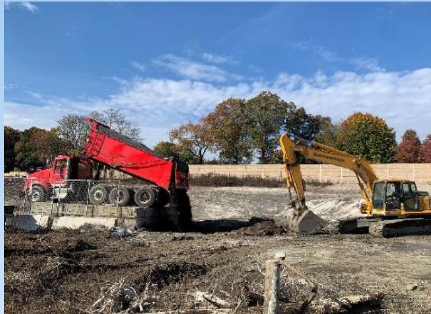
Offloading PHC soils from 250 Ferry Blvd to the TFS
