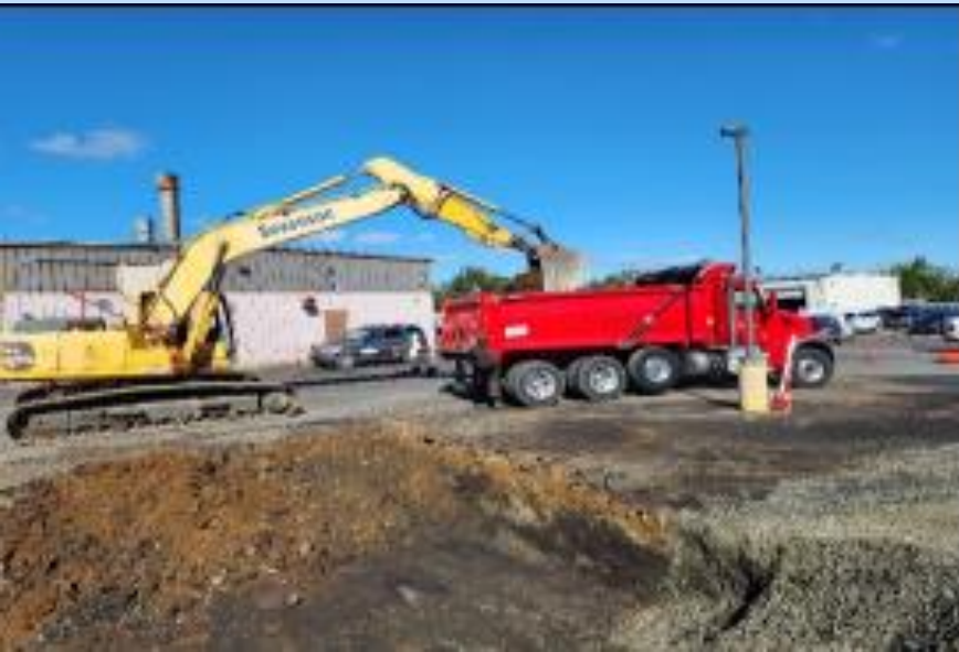
250 Ferry Blvd - Excavation
