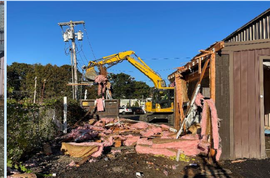
250 Ferry Blvd – Demolishing Shed
