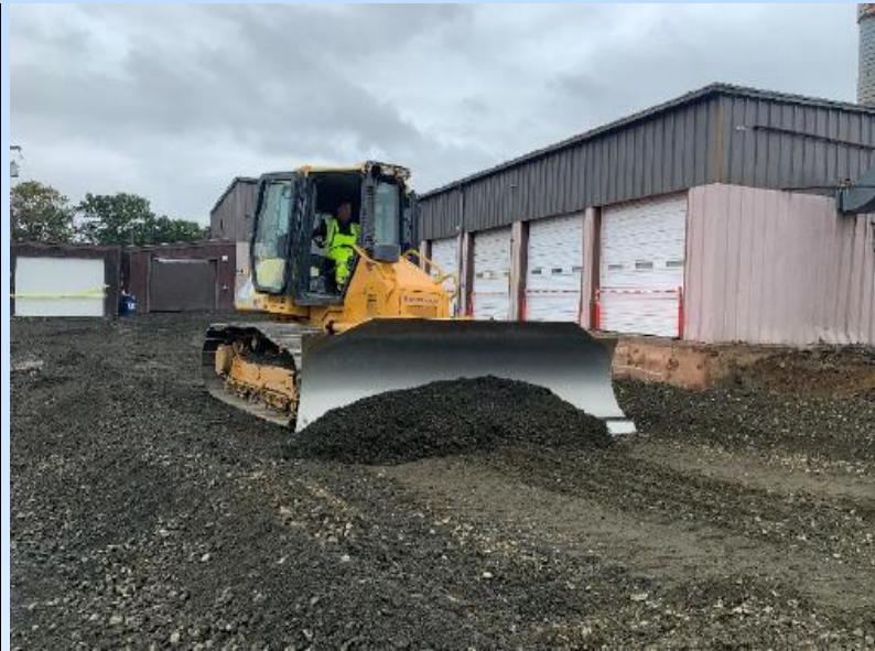
250 Ferry Blvd – Grading Backfill
