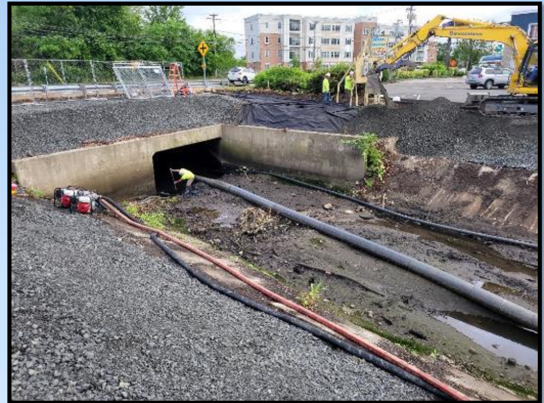
Box culvert outlet at Ferry Blvd
