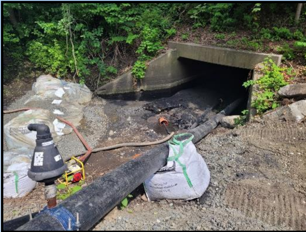
Box culvert inlet at East Broadway
