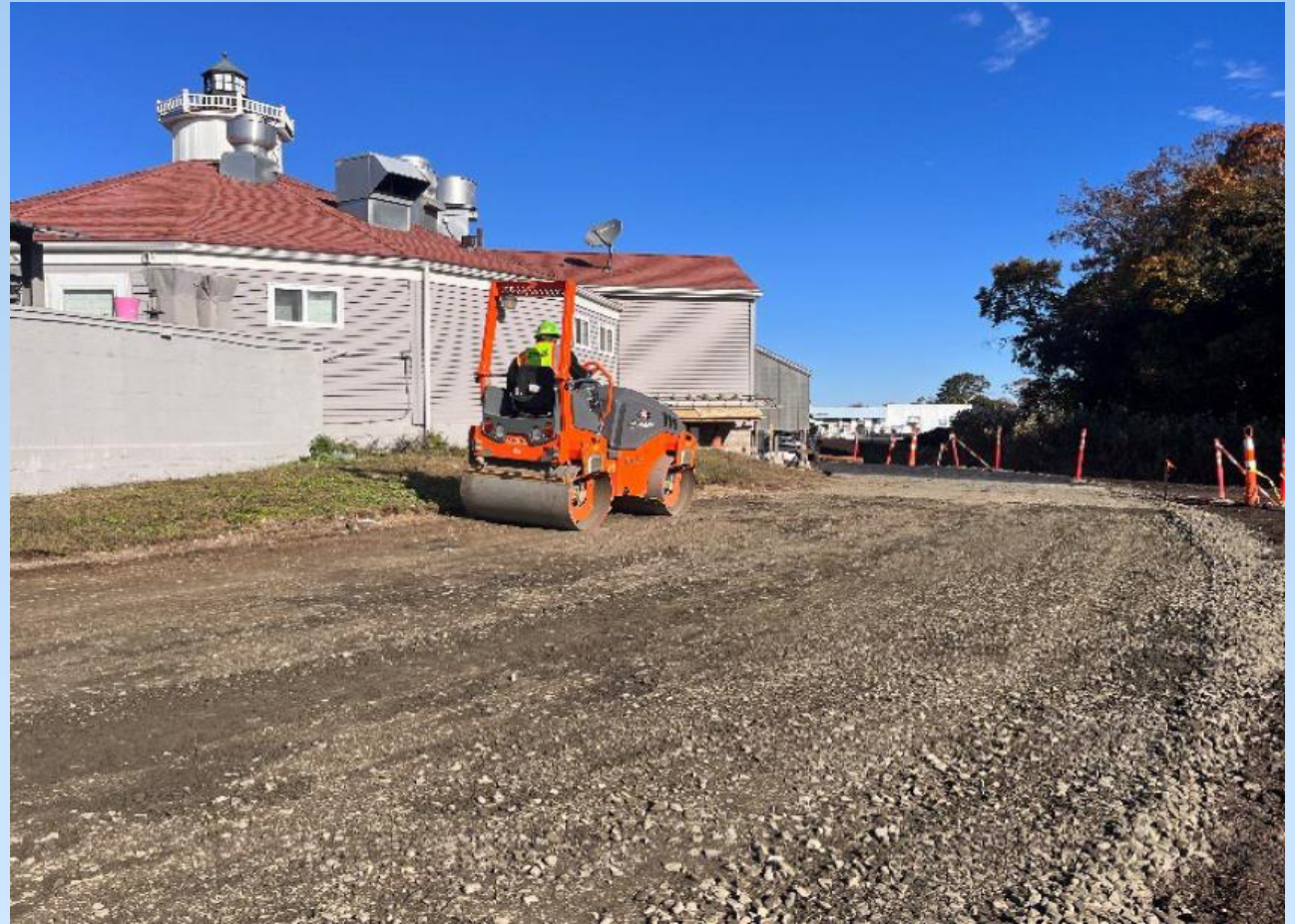
Compacting subbase to prepare for paving at 170 Ferry Blvd
