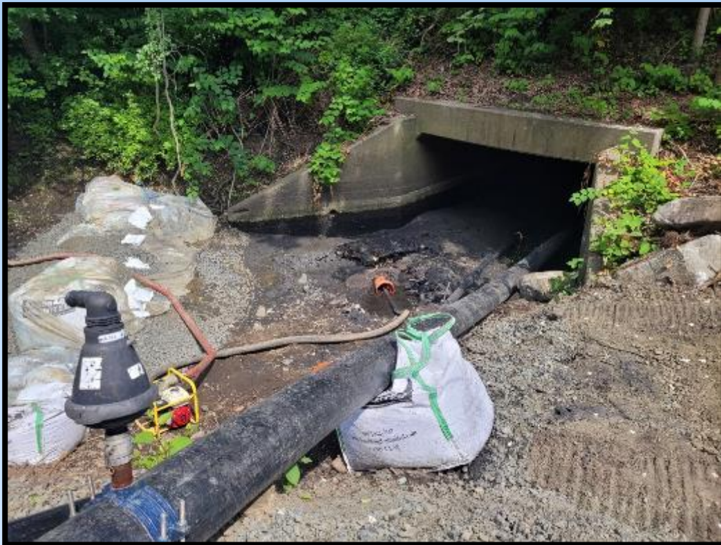
Box culvert inlet at East Broadway
