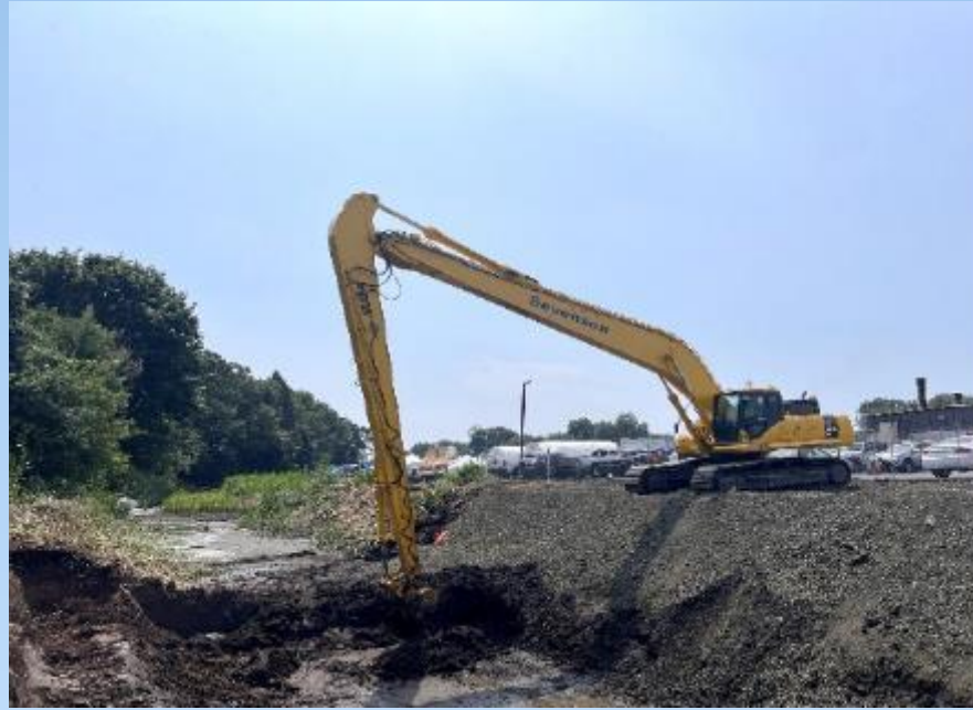
Excavating saturated Raymark Waste from Upper Ferry Creek
