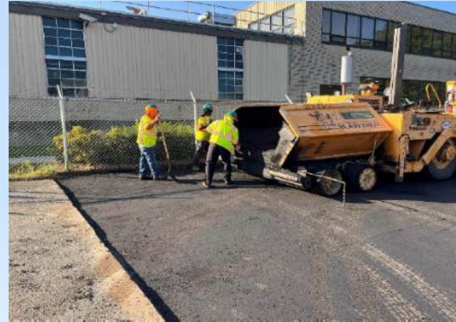
Asphalt paving Ashcroft Parking Lot
