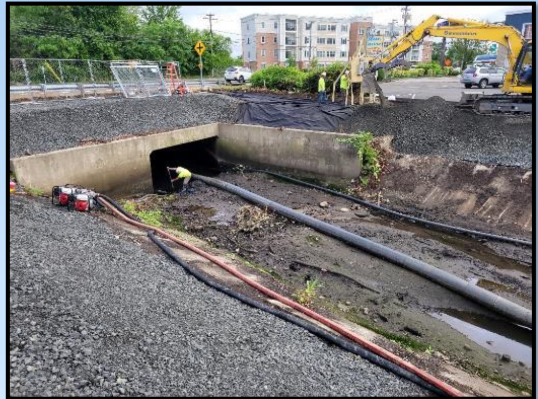
Box culvert outlet at Ferry Blvd
