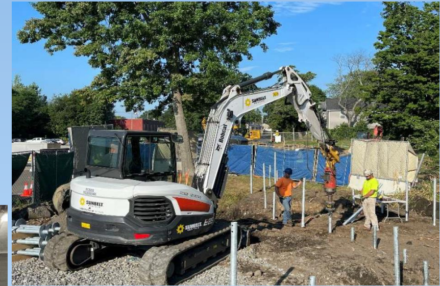
SWC Helical Piles
