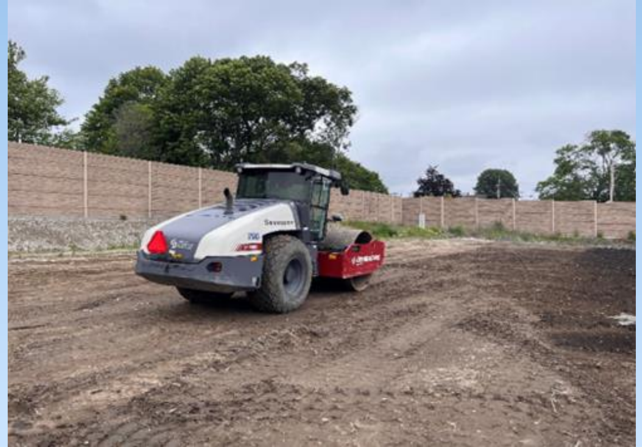
Roller Compaction
