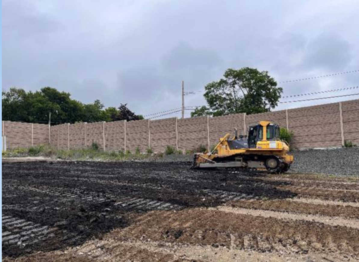
Material Grading Within OU4 Consolidation Area
