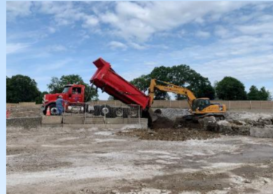
Offloading Raymark Waste for consolidation at OU4.
