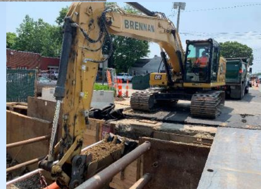
Excavating in front of 390 East Main Street to install box culverts.
