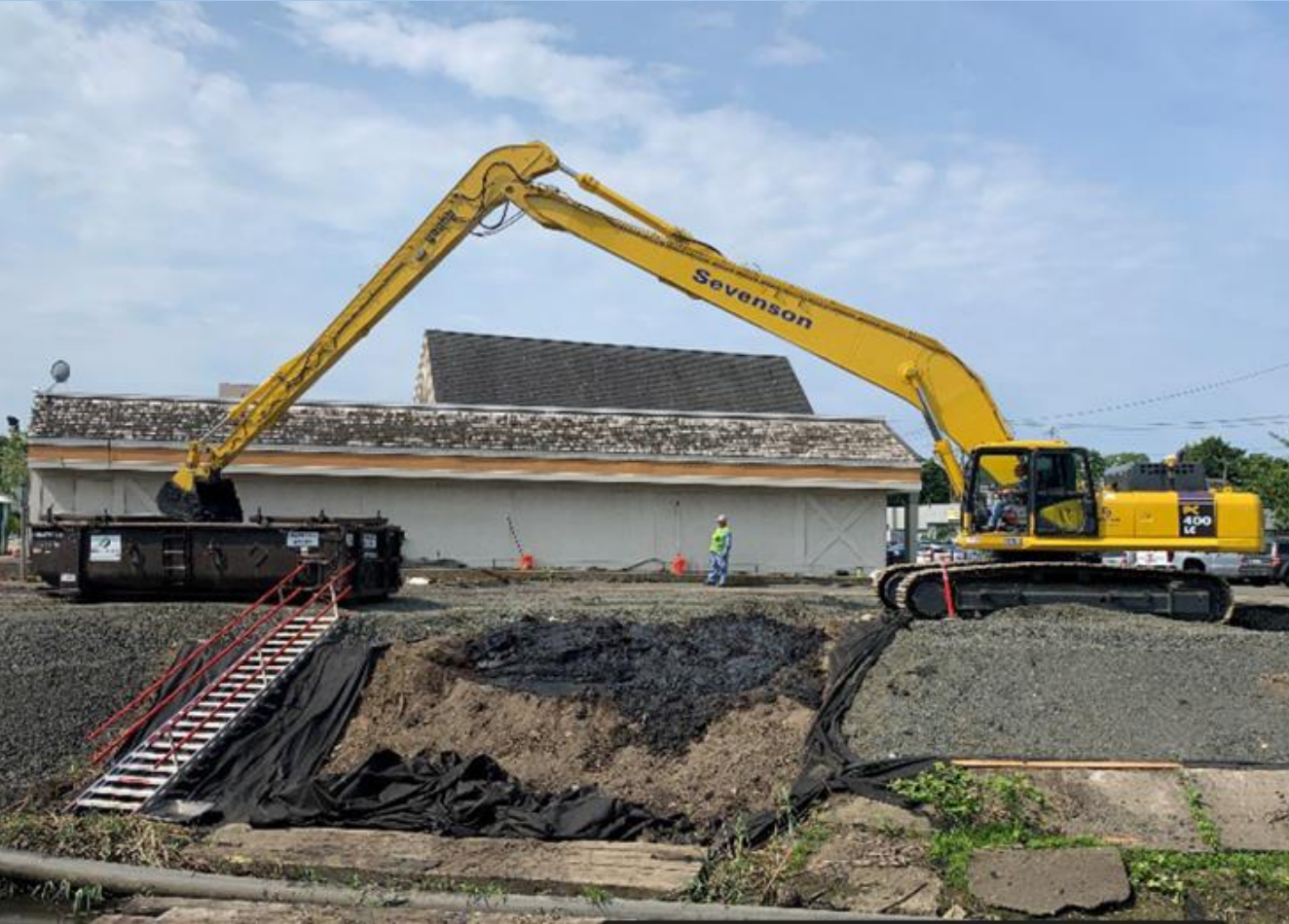
Loading Material From Ferry Creek (OU3)
