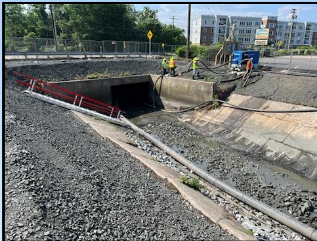
Outlet of cleaned culvert
