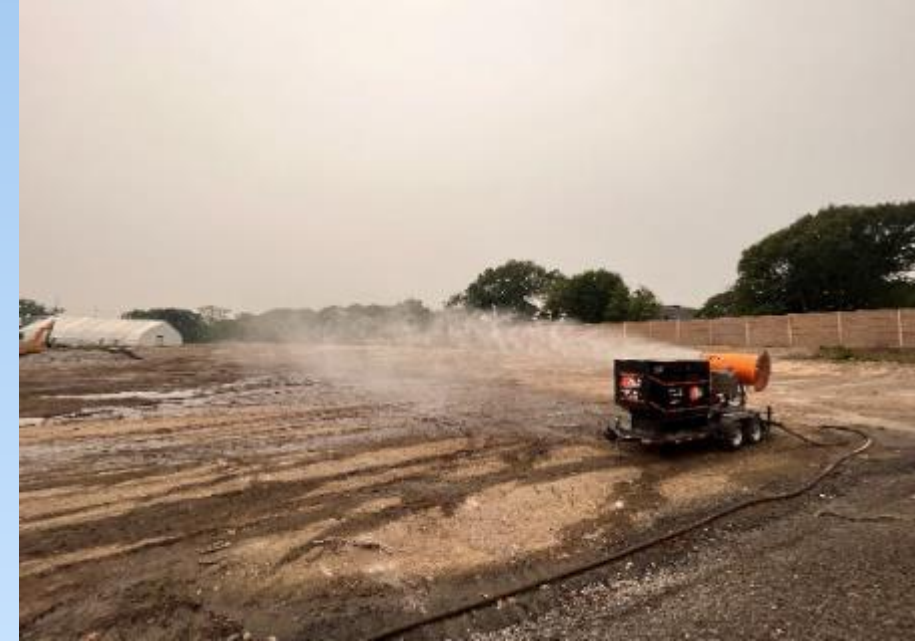
Utilizing Dustboss for dust control at OU4.
