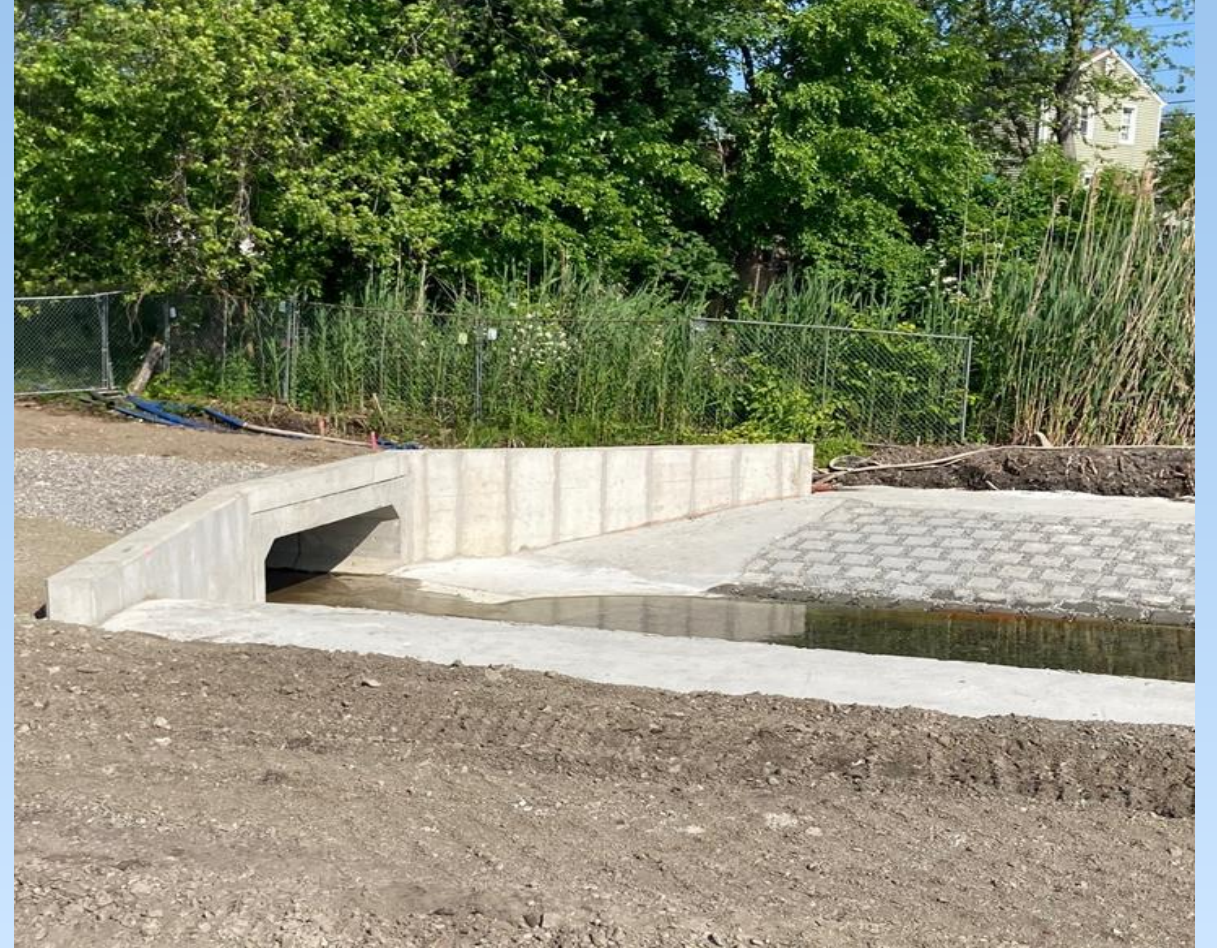
Completed Outlet and Headwall
