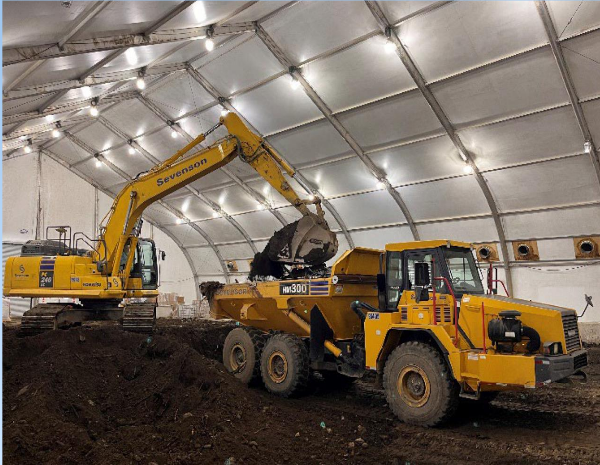
Loading Amended Soil for Consolidation
