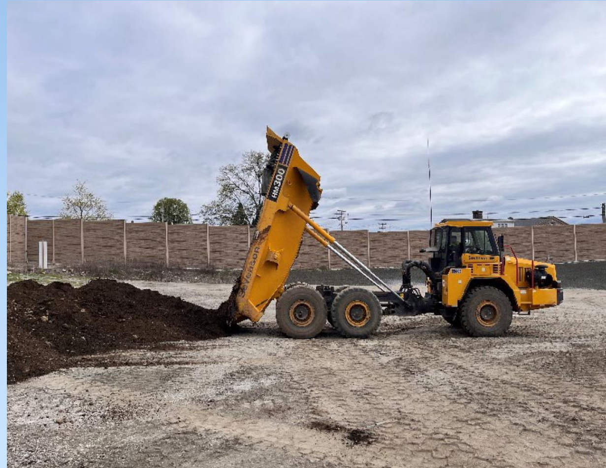
Material Placement Within OU4 Consolidation Area
