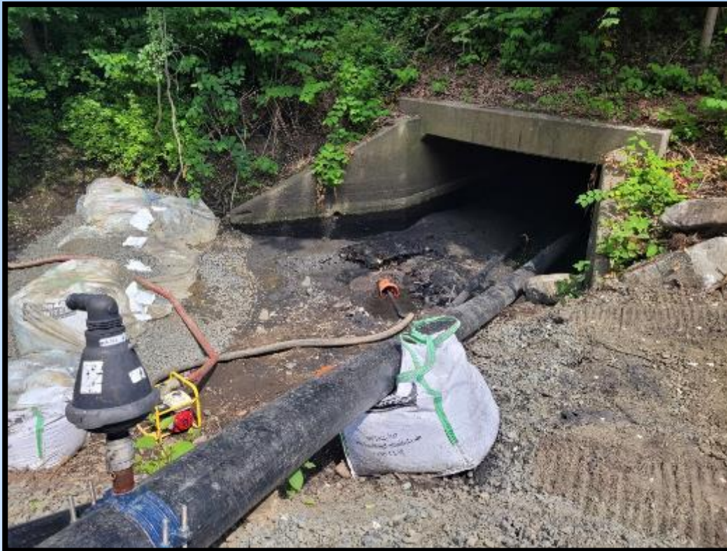
Box culvert inlet at East Broadway
