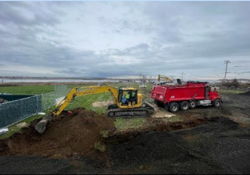
Beacon Point- Excavation
