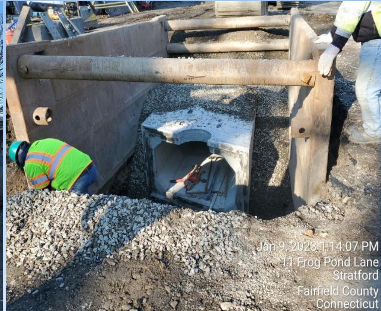
Box Culvert Installation at DPW
