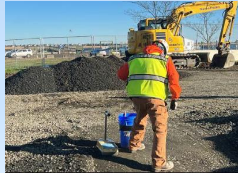
Beacon Point – Compaction Testing
