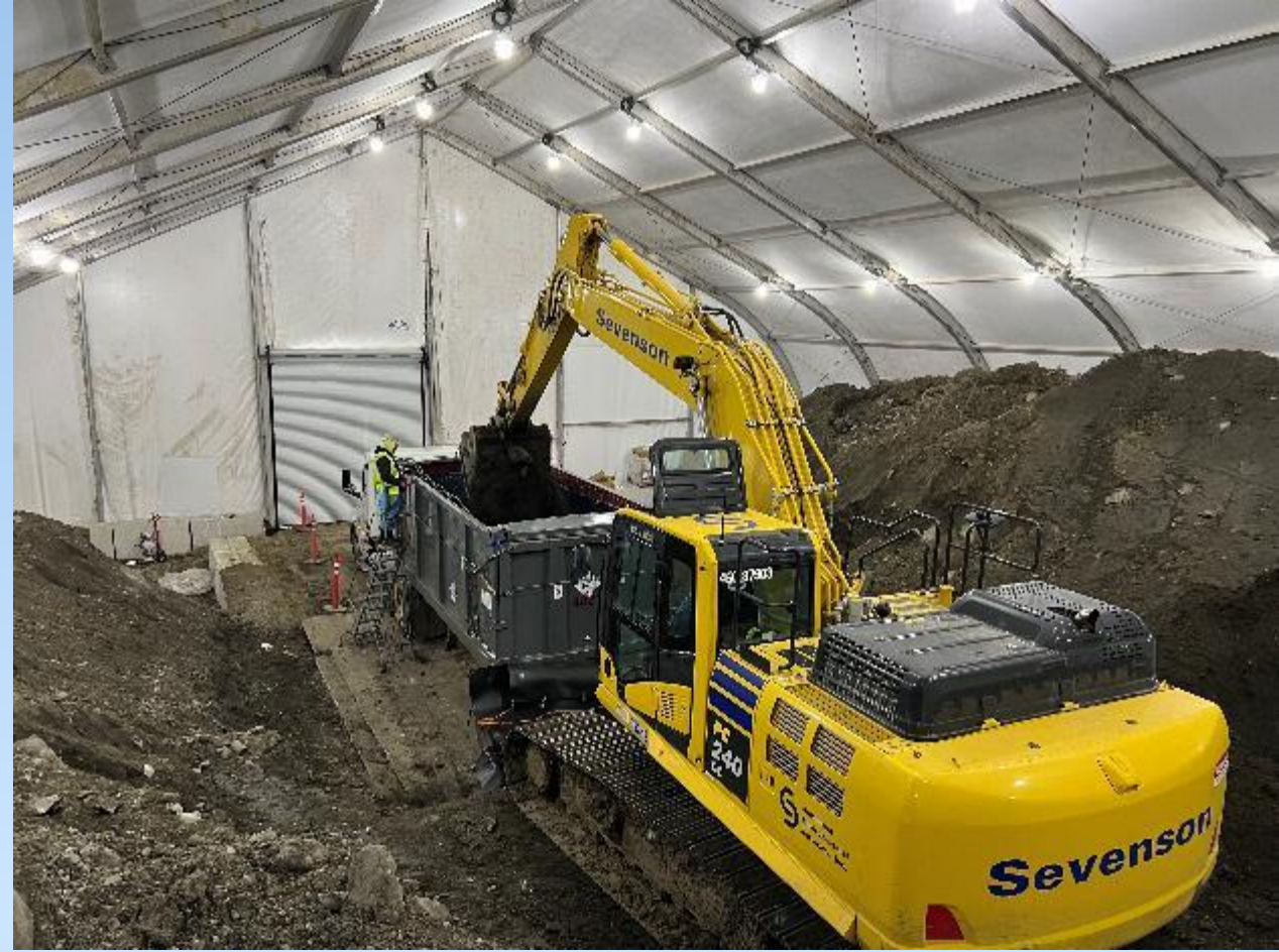
Loading PHC Material for Off-Site Disposal
