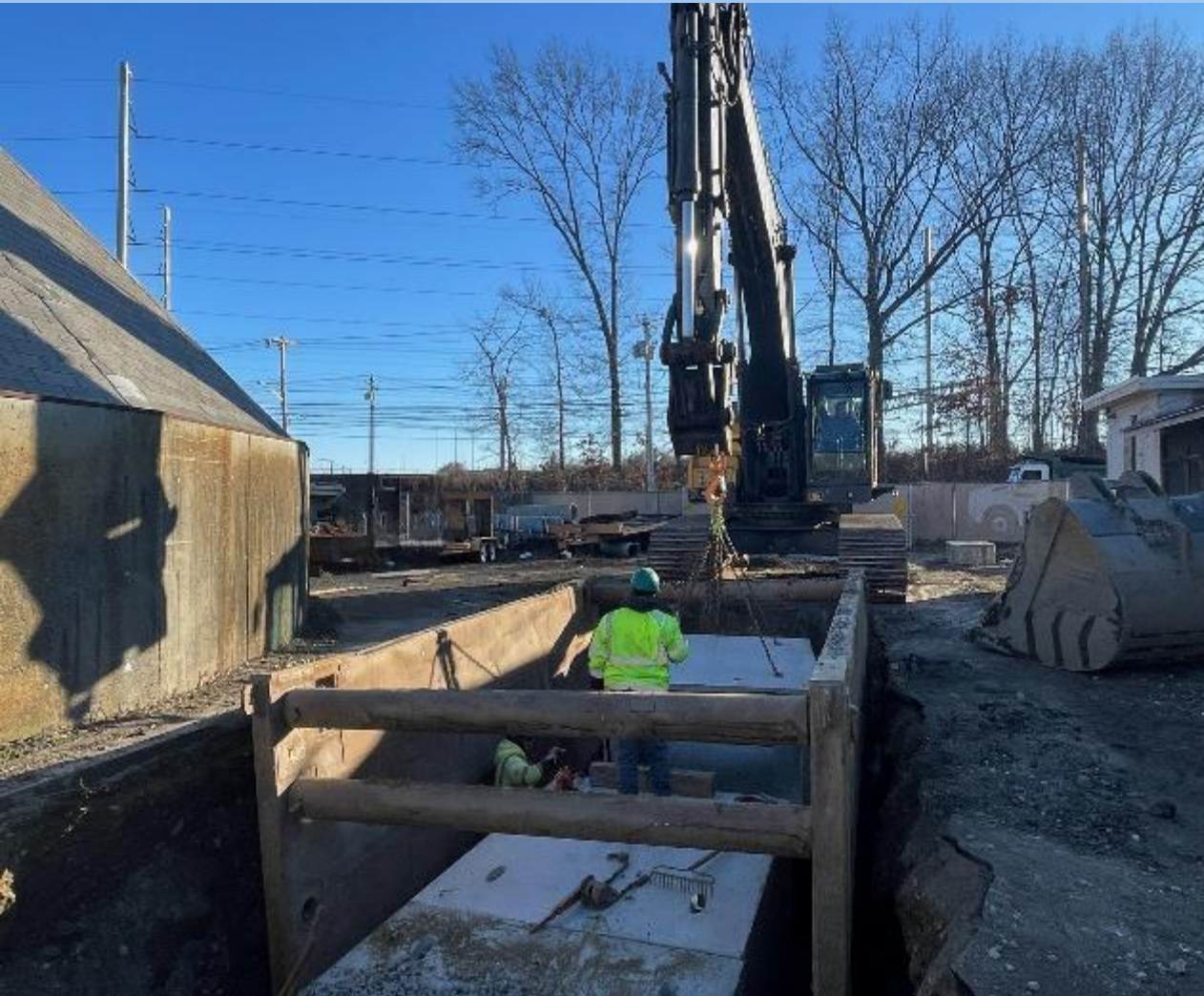
Box Culvert Installation at DPW
