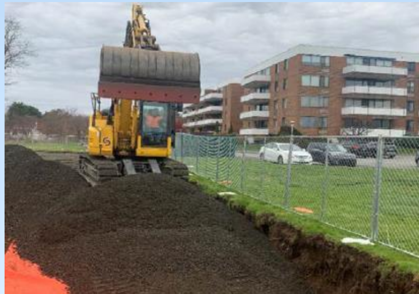
Beacon Point- Placing Clean Fill
