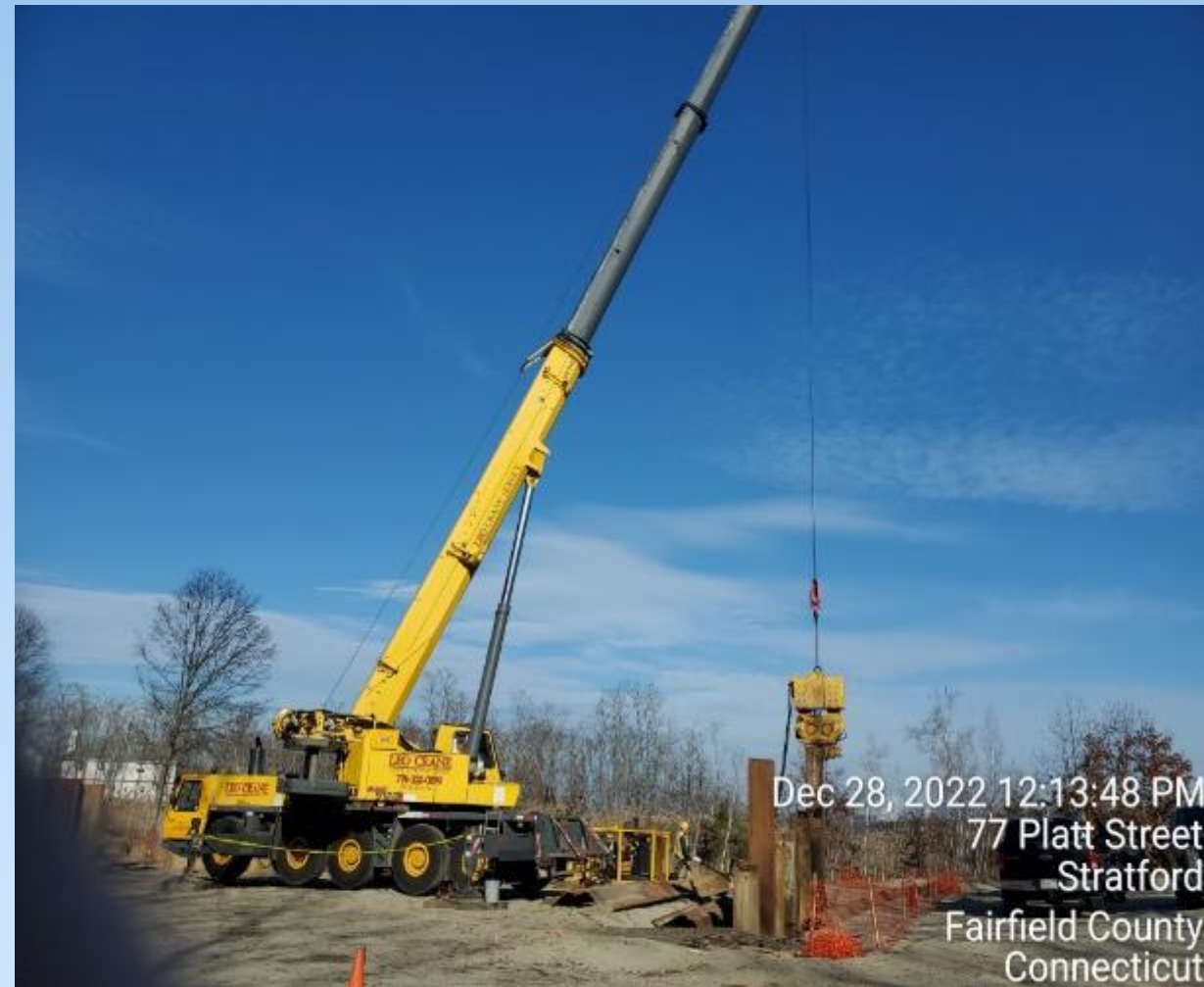
Sheet pile installation
