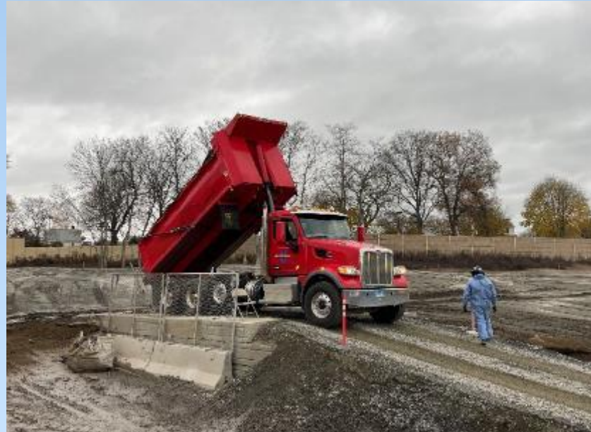
Loading PHC soils for offsite disposal within the TFS at OU4
