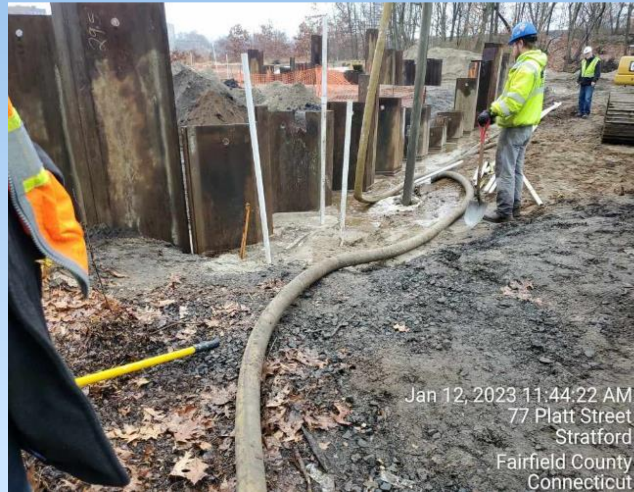
Dewatering well point installation
