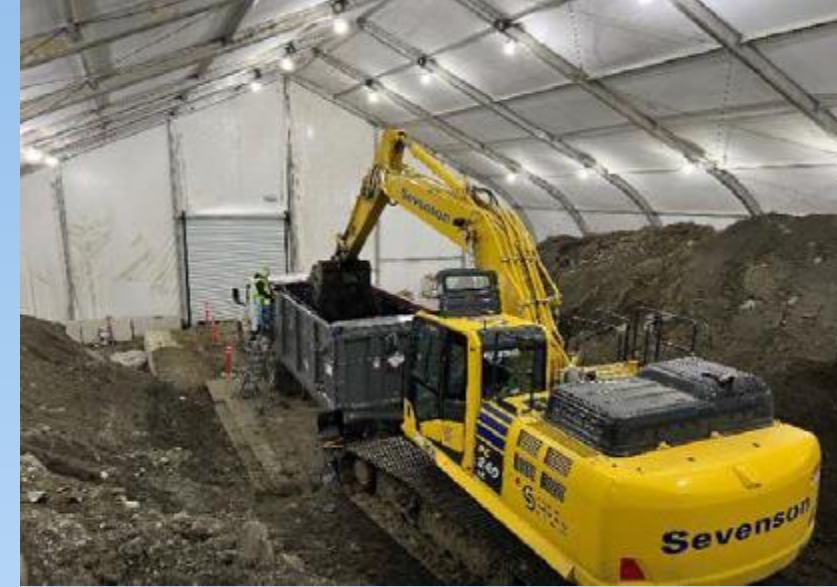
Offloading Raymark Waste at OU4 Consolidation Area
