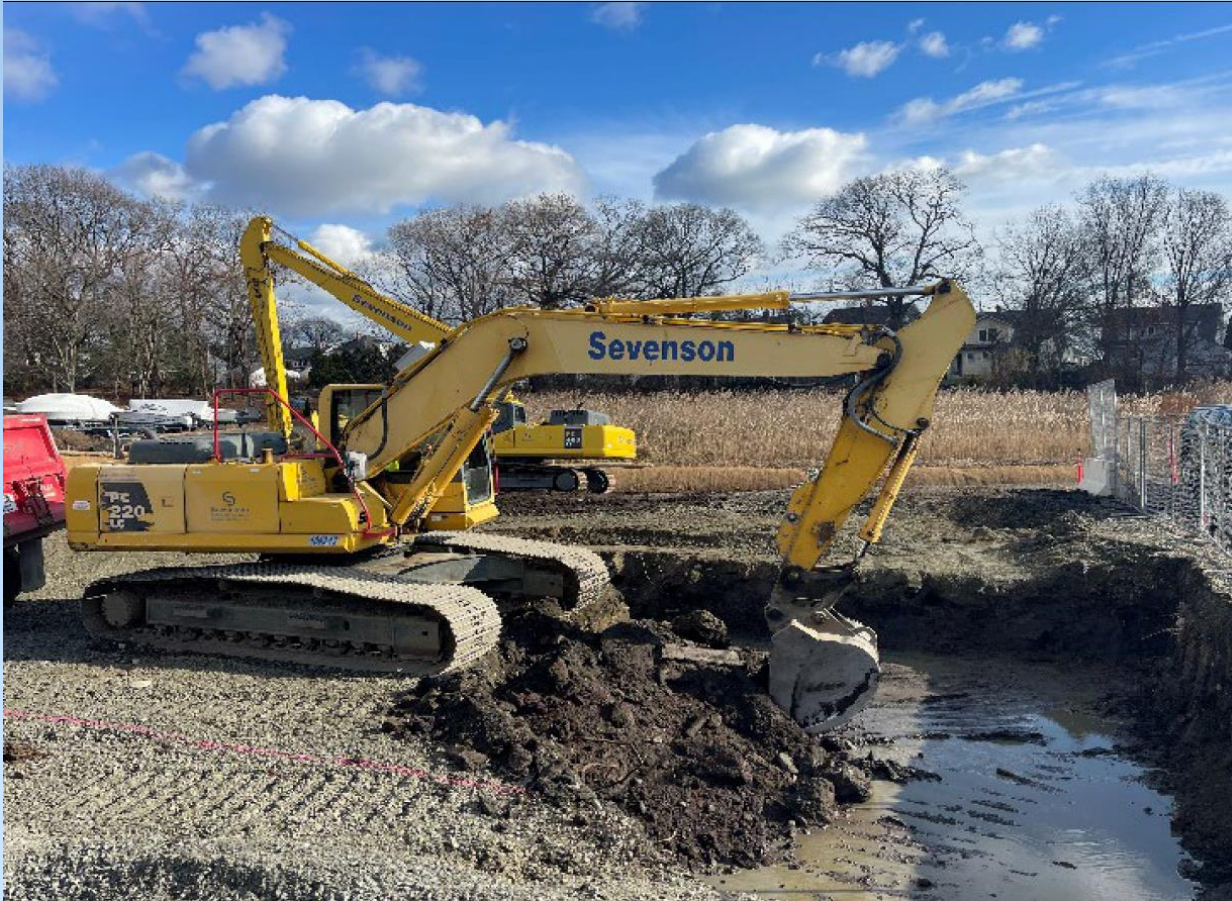
Excavating Raymark Waste at 300 Ferry Blvd
