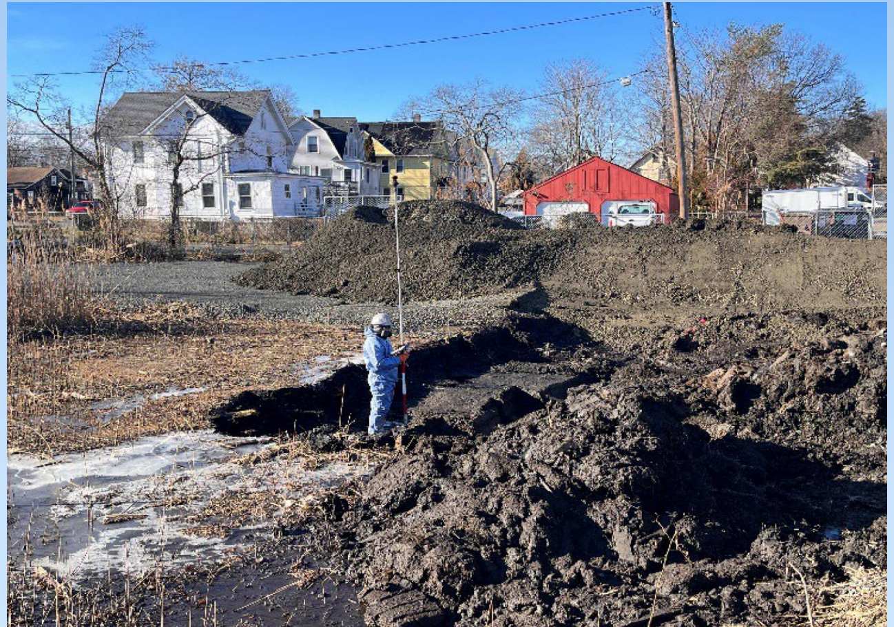
Surveyor verifying excavation depth at Lockwood Avenue property
