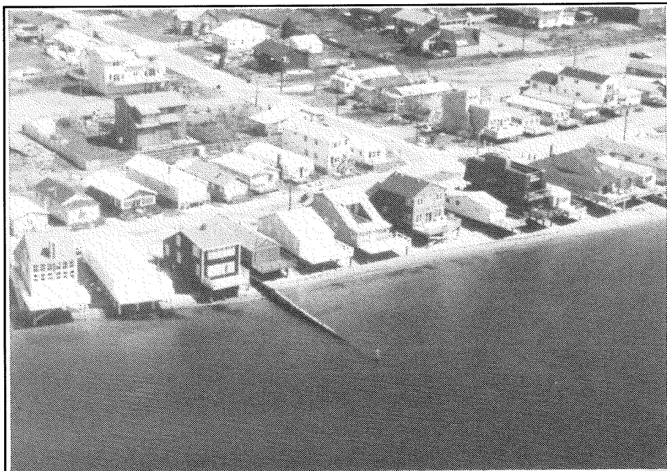
Figure 5-11: Beach Cottage Area.
