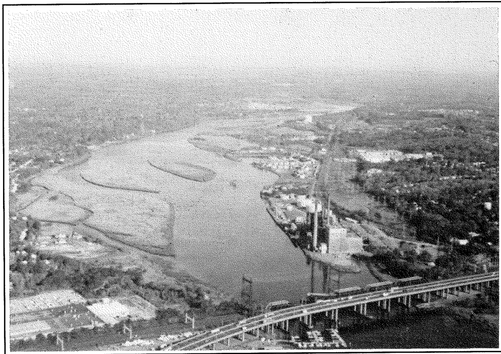
Figure 1-4: Upper Housatonic River Management Area looking north; I-95, railroad bridge, and Devon Power Station in foreground.
