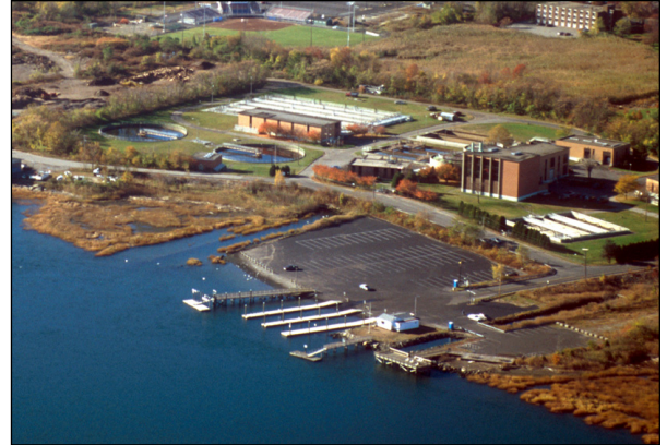
Aerial View of Birdseye Boat Launch Area
