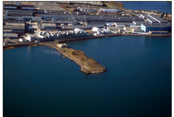
Aerial View of Jetty at Army Engine Plant
