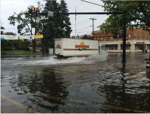
Street flooding in downtown Fairfield immediately downgradient from impervious surfaces
