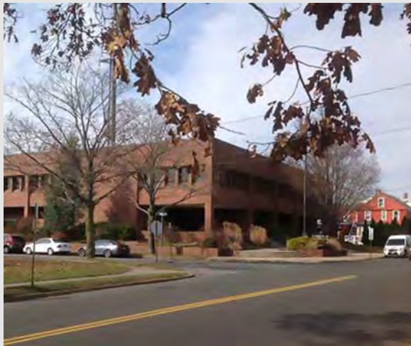
Fairfield microgrid area; photo by Schneider Electric Blog
