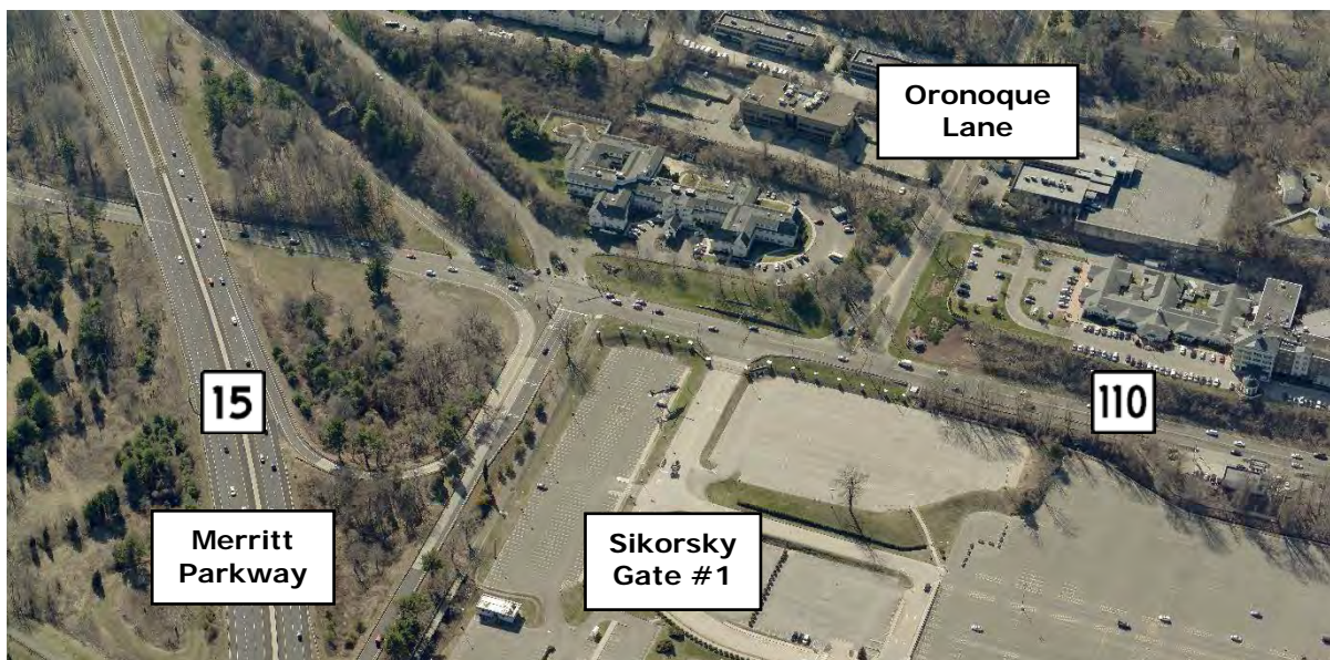
Route 110 from Merritt Parkway to Oronoque Lane – Looking West
