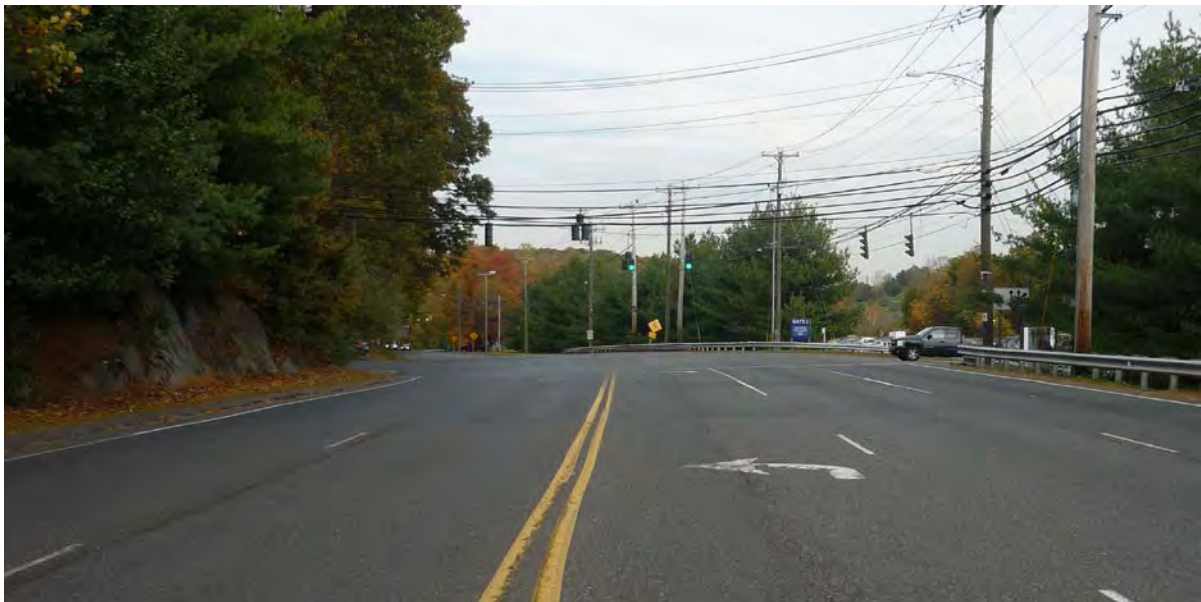
Alignment of Route 110 at Warner Hill Road/Sikorsky Gate #2 – Looking North
