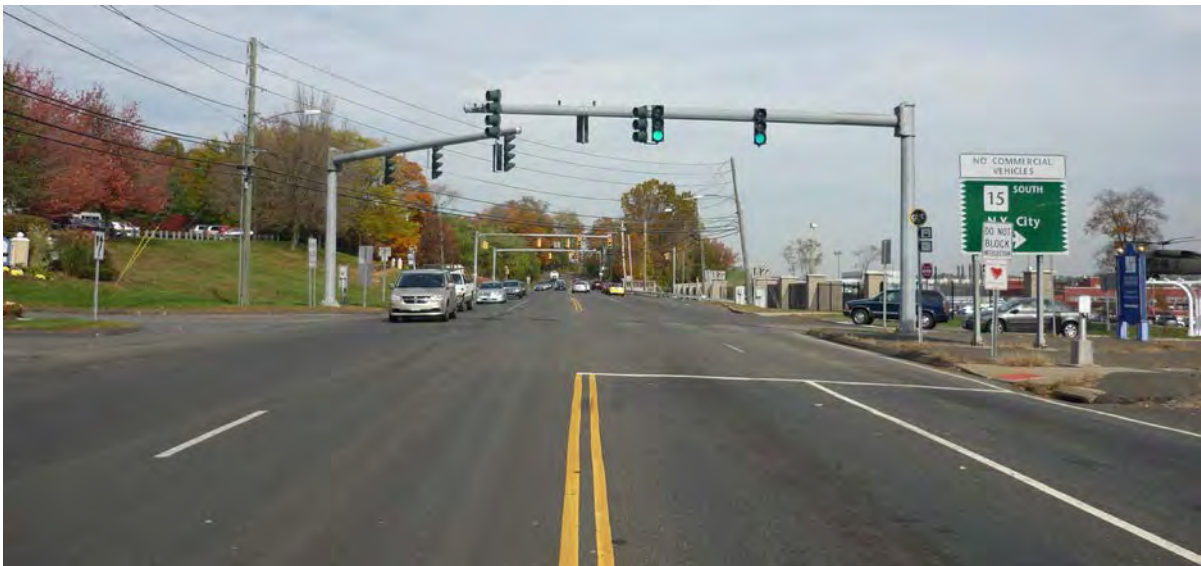
Route 110 at Merritt Parkway Southbound Ramps – Looking North
