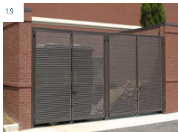
Picture to the top: Example of recommended screening of trash containers to prevent views from surrounding streets.
