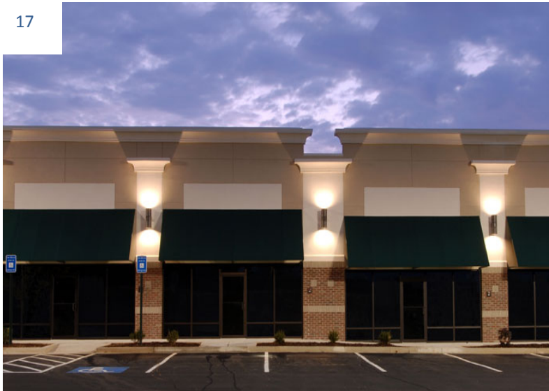
Picture to the top: Example of recommended light fixtures' positioning to reduce or limit glare.
