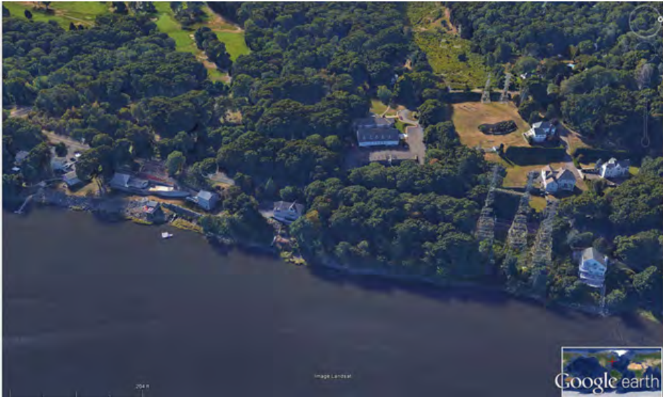
Image 26: Shoreline representative of area along River Road. Houses located at top of embankment, at approximately Elevation 20 to 30 feet NAVD88. Power line crossing at right side of image.
