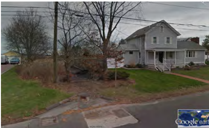
Image 21: Drainage swale and stormwater catch basins at Elm Street, discharging to tidal wetlands and hydraulically connected to the Housatonic River.
