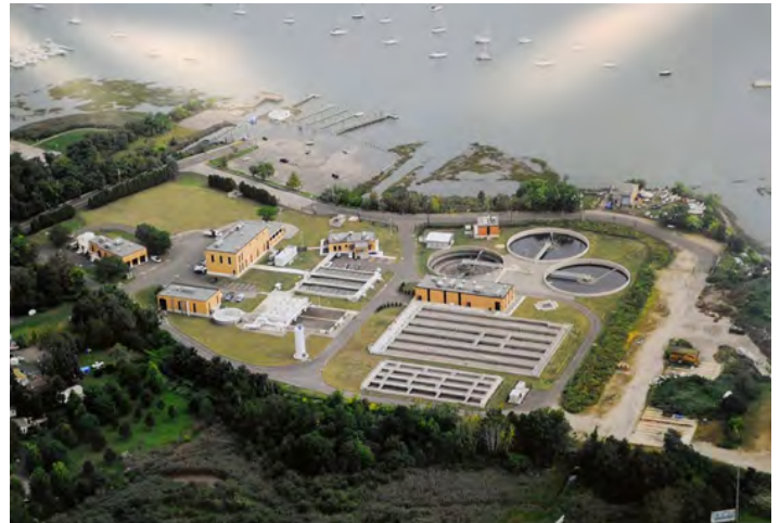
Lifeline Facilities: Sanitary Sewer Stratford Water Pollution Control Facility (Credit: CTPOST)
