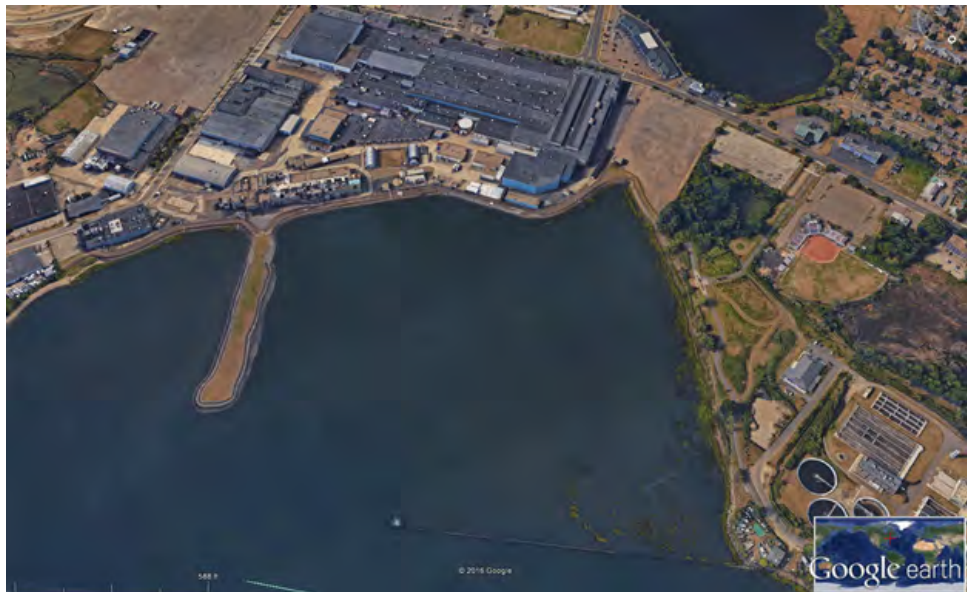
Image 13: The shoreline in front of the Stratford Army Engine Plant is protected with a levee with a crest elevation of 9 to 10 feet NAVD88 and a rock revetment shoreline protection. An area of sheltered water has been created in front of the Stratford Army Engine Plant by an approximately 1,200-foot long rock breakwater (extending southeast from the wastewater treatment plant) and an approximately 800-foot long, earthen-filled jetty. This area has significantly filled with sediment.
