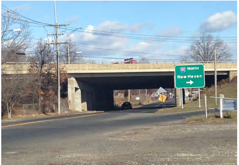
Surf Avenue Underpass
