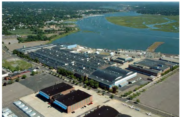
Hazardous Materials Facilities Stratford Army Engine Plant (Credit: Hearst CT News 2013)
