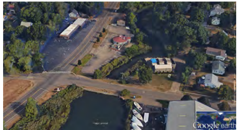
Image 22: Broad Street Bridge over Ferry Creek. Bridge includes box culvert and tide gate, with pump station to discharge river flow during coastal storms. New bridge currently proposed. Existing bridge deck at approximately Elevation 6 feet NAVD88.
