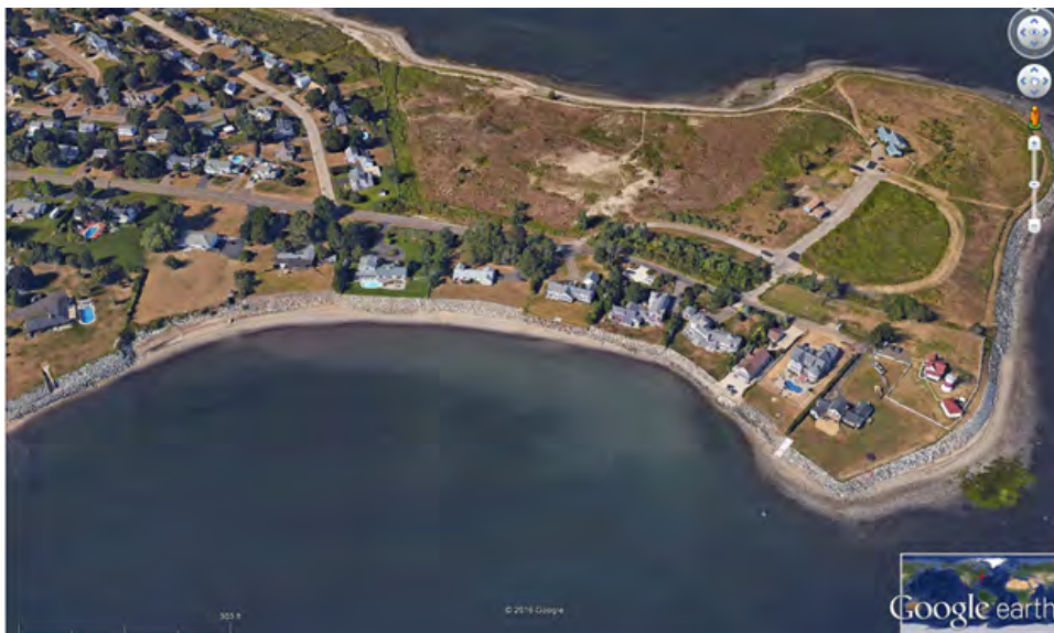
Image 8: Typical representation of quarry stone revetment shore protection along Lordship Beach and Stratford Point.
