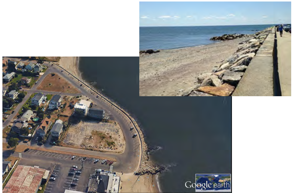
Image 6: An approximately 900-foot long stone seawall and quarry stone revetment are present along the southern side of Beach Drive. Detail photo of wall, revetment and beach.
