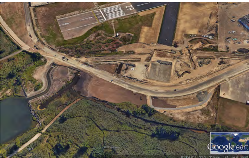
Image 11: Hydraulic connection of the Marine Basin to the tidal wetland areas surrounding the Sikorsky Memorial Airport via culverts constructed beneath the recently reconstructed section of Lordship Boulevard.
