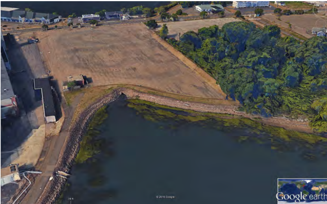
Image 16: Limits of the Stratford Army Engine Plant levee. As shown above, the levee winds around existing parking area. The image also shows the drainage culvert that hydraulically connects Frash Pond to the Housatonic River.
