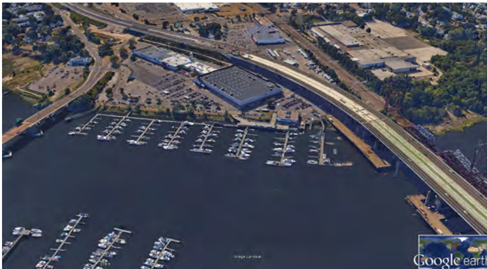
Image 24: Route 1, Interstate 95 and Amtrak river crossings. Retail center at approximately Elevation 10 feet NAVD88.
