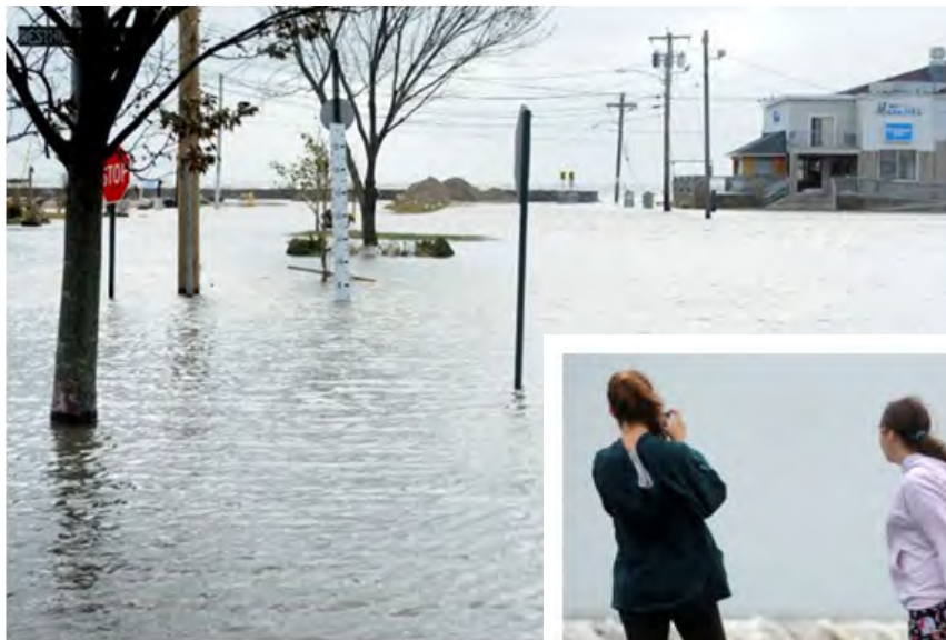
Flooding in Lordship neighborhood during Hurricane Sandy (Source: ctpost.com)
