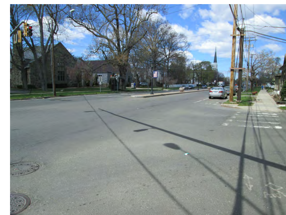
STA. 7+75 LOOKING NORTH
