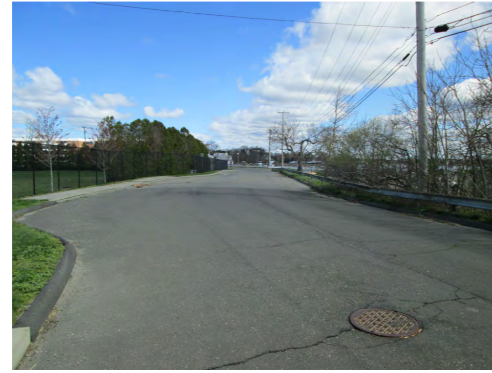
STA. 7+50 LOOKING NORTH
