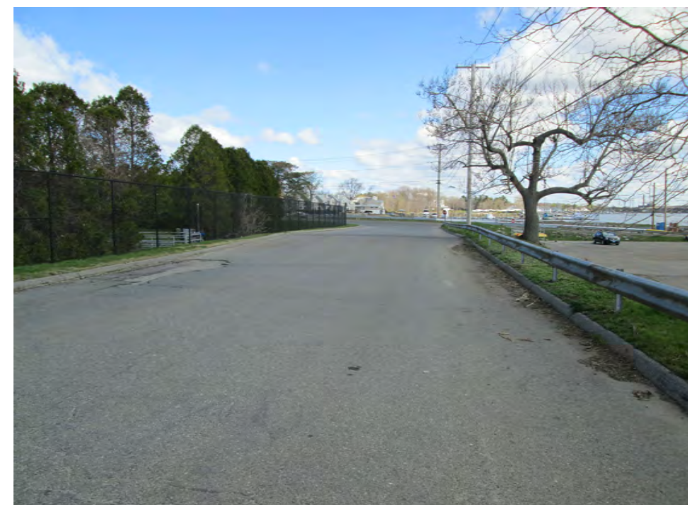
STA. 8+50 LOOKING NORTH
