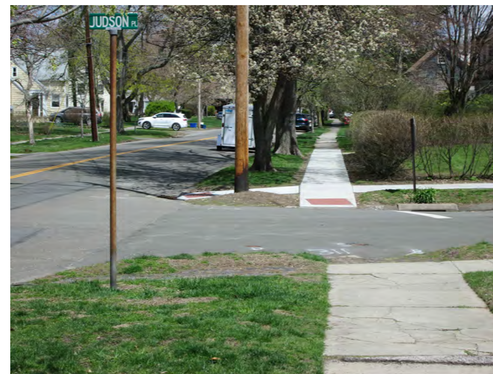
STA. 58+25 LOOKING NORTHEAST
