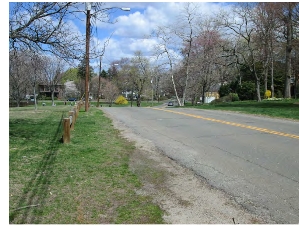
STA. 50+50 LOOKING NORTH
