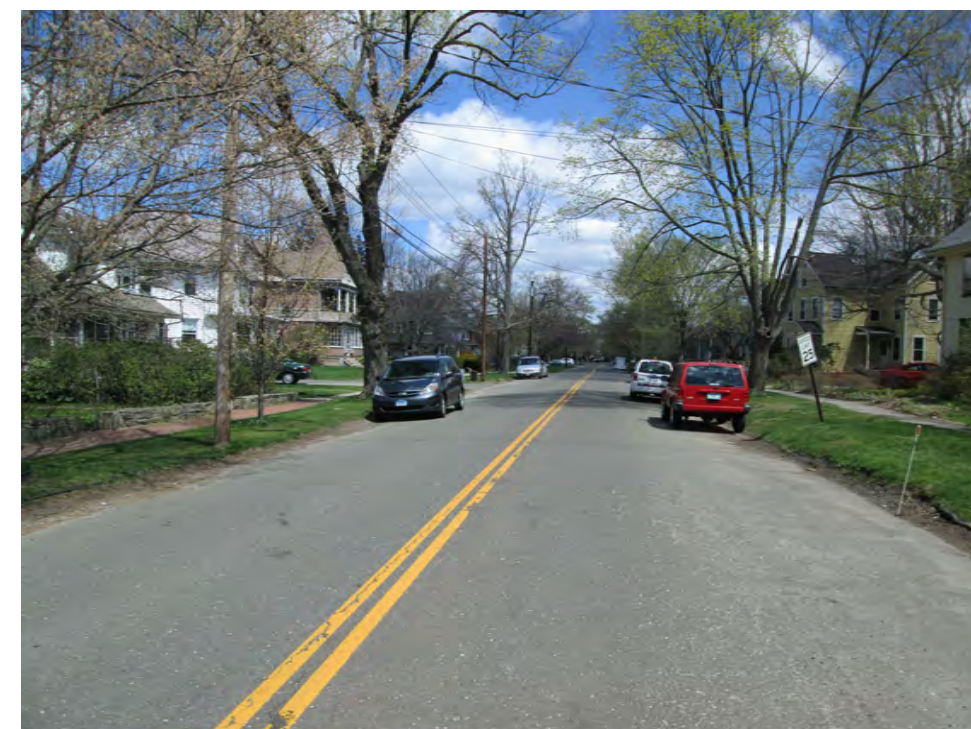
STA. 57+75 LOOKING NORTHEAST
