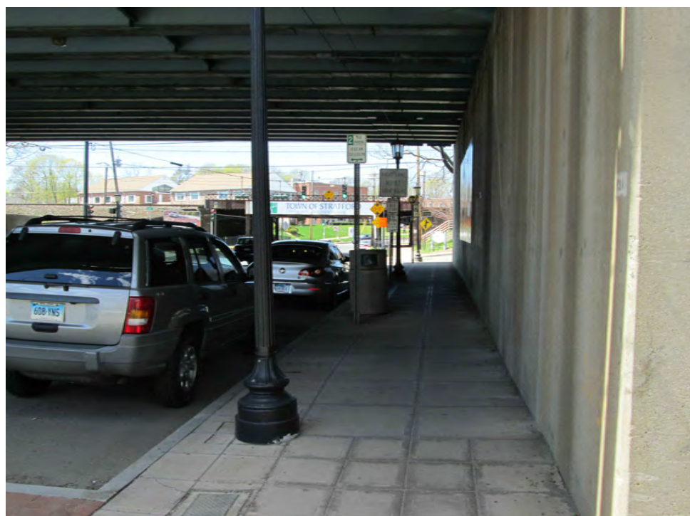
STA. 87+00 LOOKING NORTHWEST
