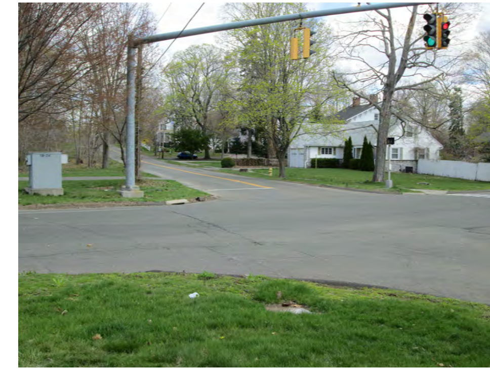
STA. 43+50 LOOKING NORTH
