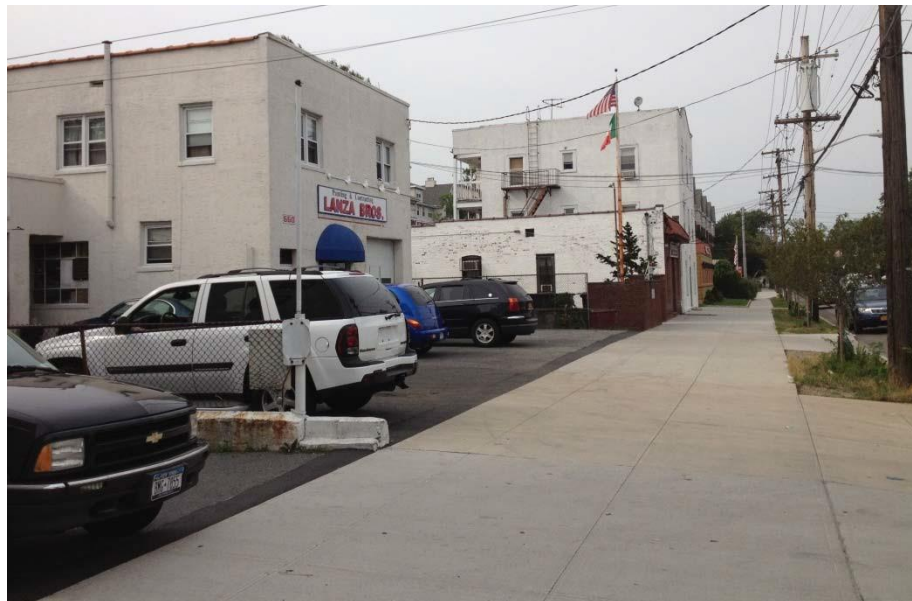
BELOW: Parking between buildings and the street disrupts the pedestrian experience, and is discouraged.
