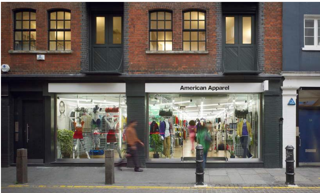
The windows at top are obstructed by signage or display items, detracting from the streetscape, which should be avoided. The windows at the bottom are open and inviting to the pedestrian.
