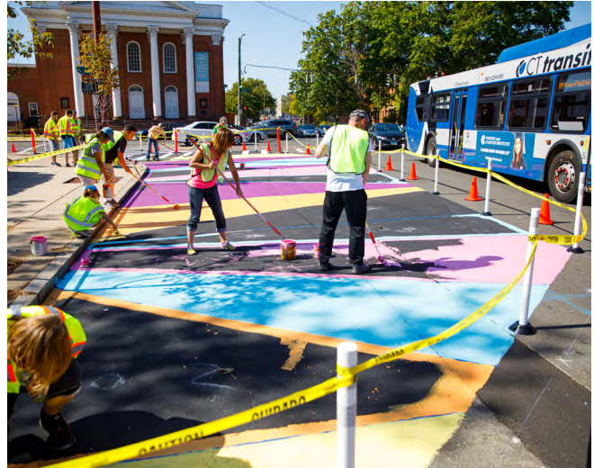
Example of tactical urbanism creation in Downtown Hartford. A wide intersection was colorfully painted to provide more room for pedestrians while also helping to reduce vehicular speeds.
