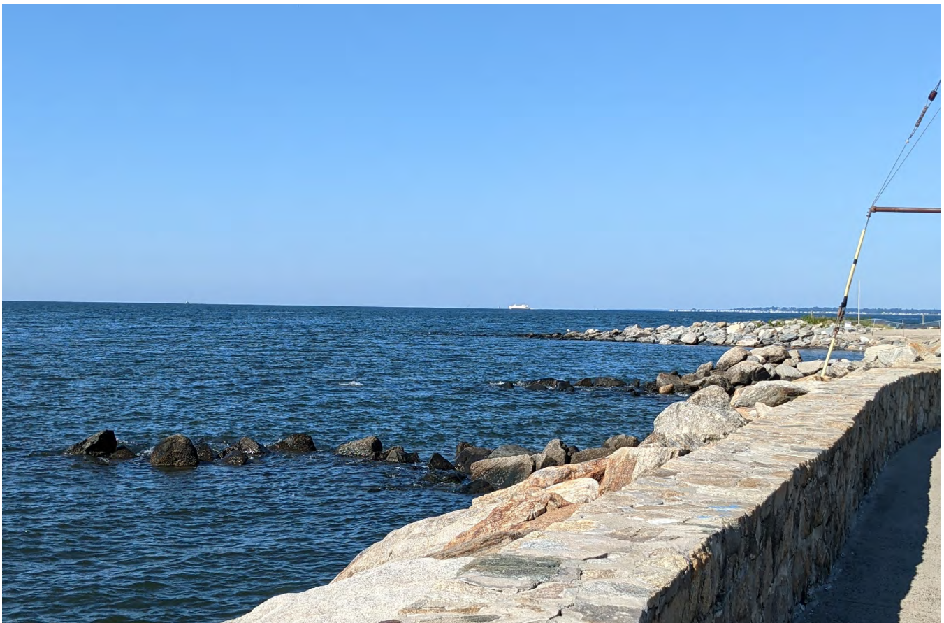
Seawall in Lordship neighborhood
