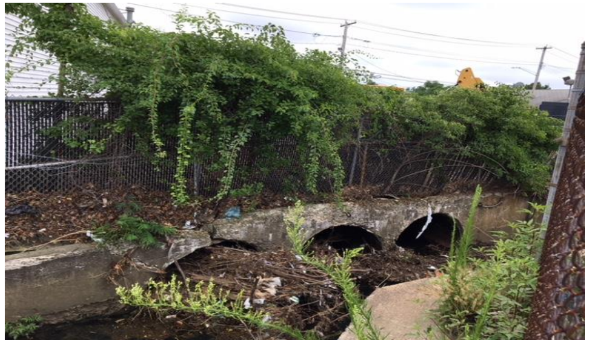
This photo of Bruce Brook shows a significantly damaged concrete headwall and clogged culvert pipes caused by debris.
